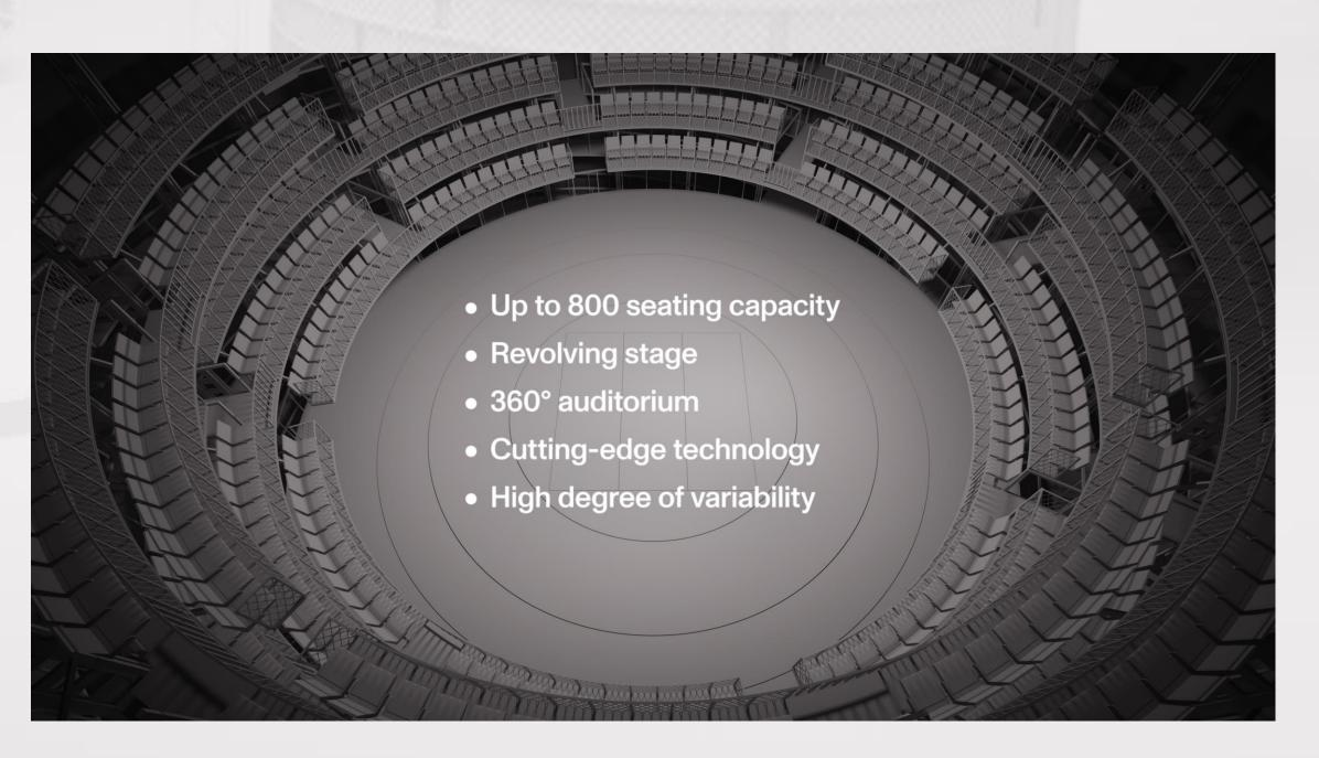
There a system of concentrical stage turntables. Outer with 13,8m diameter and inner with 9m diameter.
